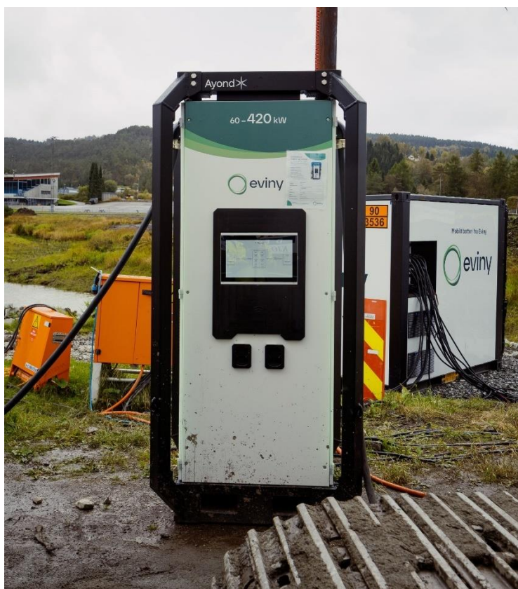
Figur 6; Eviny hurtiglader 60-420kW CCS - "Eviny"
